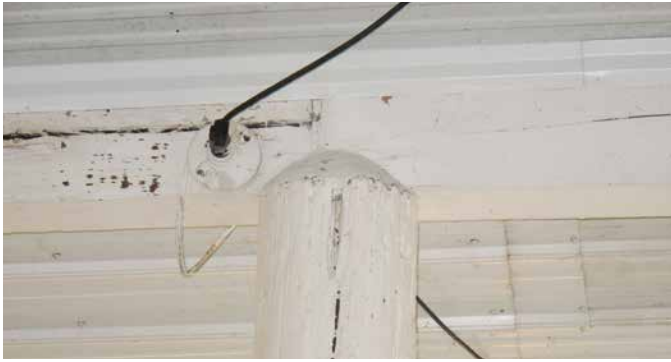
Steep-sided pyramids of cement on top of beams dissuade birds from making nests.
