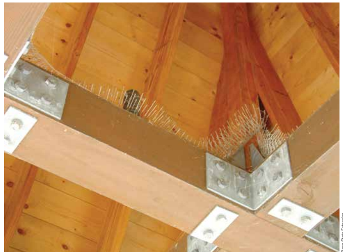
Use bird spikes to prevent nesting and/or place plastic over exposed produce areas.
