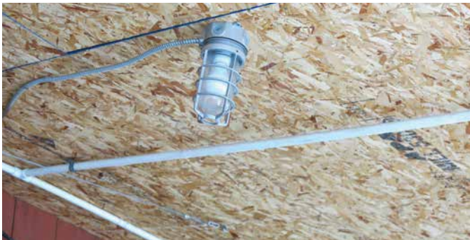
Covering the ceiling in the packhouse with plywood is one way to keep birds out of rafters. Lightbulbs should be shatterproof or covered with shatterproof materials.
