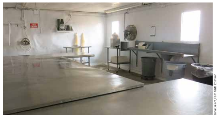
Stainless steel and washable walls, while not always feasible, are important in packhouses such as this one that grows and packages sprouts.
