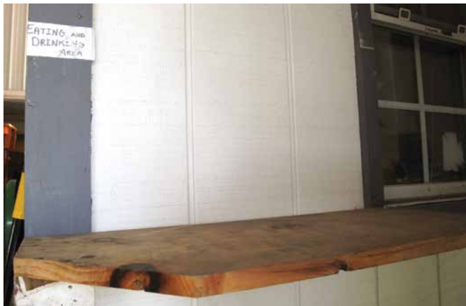
Designate a separate area for eating and drinking. For example, here the farmer has a specific shelf in another area of the building for water bottles.
