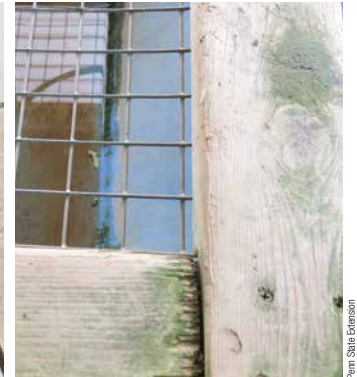
Unsealed wood surfaces that come into contact with produce, such as this screen table, are not recommended. Pathogens may multiply in the cracks.
