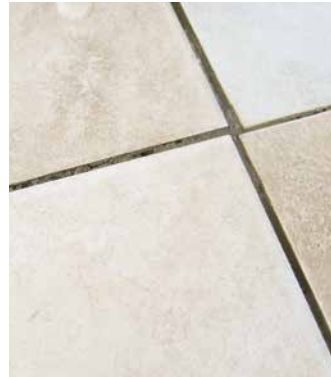
The grout in this tile countertop used in a wash station can harbor pathogens. Use surfaces that can be thoroughly cleaned.
